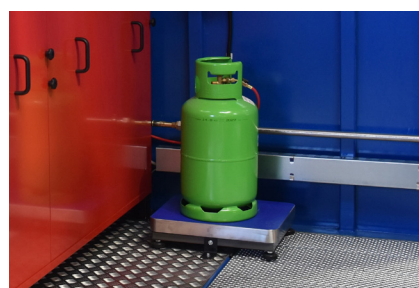
Scales accurately measure the extracted gasses
